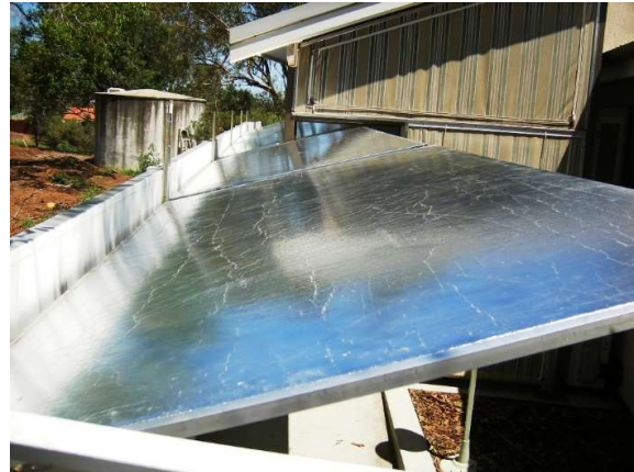
Panels set for summer shade reflect the sun to the southern sky.
