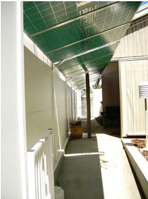
Panels, when raised in summer, shade the courtyard wall and path.
