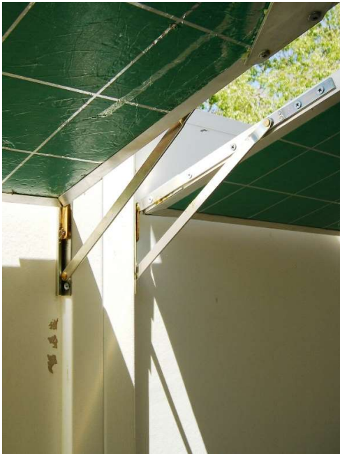
These window-stay hinges are set to support both panels to give summer shade.
