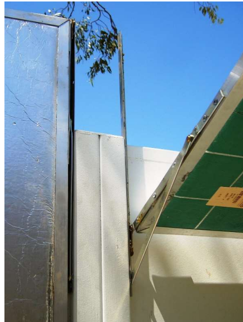
These window-stay hinges are set to support panels for winter warmth on the left, and for summer shade on the right.
